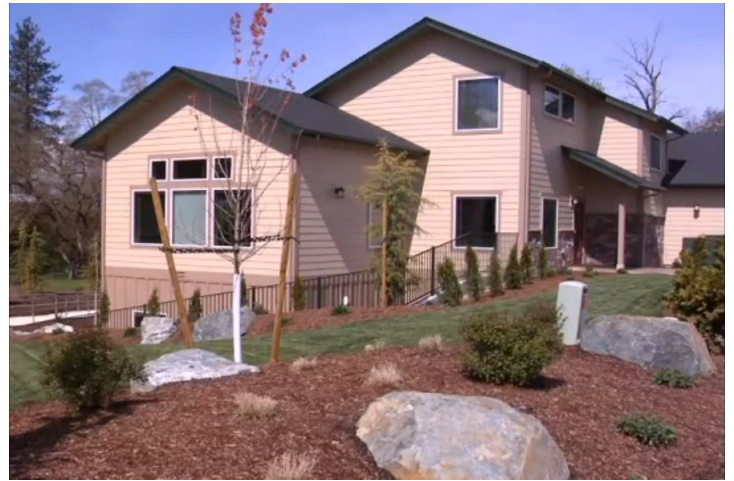
Community Services Building
